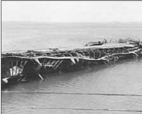
Neptunia and damaged wharf
