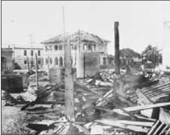
Destroyed and damaged buildings
