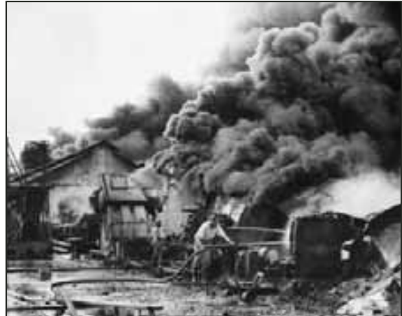
Firefighters try to extinguish the fire after bombing of naval yards
